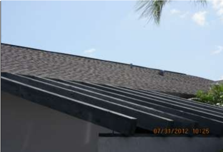
Front Elevation Asphalt-Fiberglass Shingles - No Sagging
