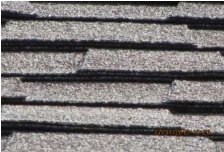
Asphalt-Fiberglass Shingled Roof No noticeable loss of Granules
