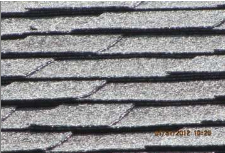
Asphalt-Fiberglass Shingled Roof No Curling or Deterioration
