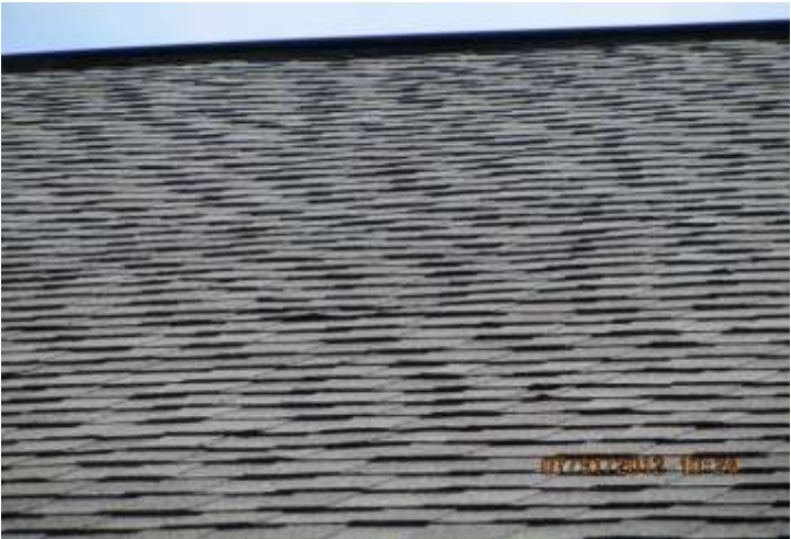
Roof Field Asphalt-Fiberglass Shingles - No Sagging
