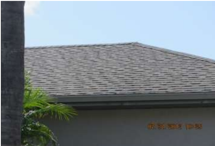
Roof Field Asphalt-Fiberglass Shingles - No Sagging
