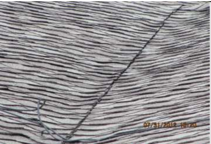
Roof Valley Asphalt-Fiberglass Shingles - Closed Flashing
